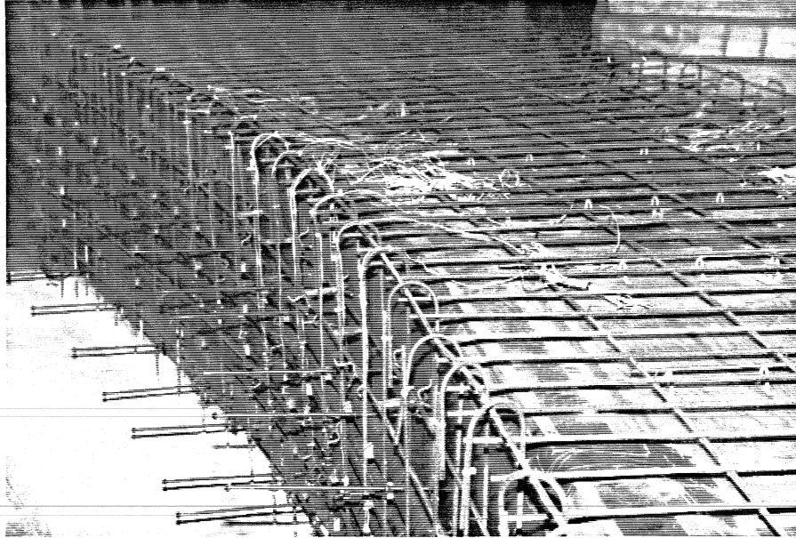
Figure 3.8 Top Slab Reinforcement
